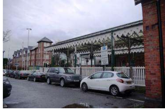
View of the east platform looking north
