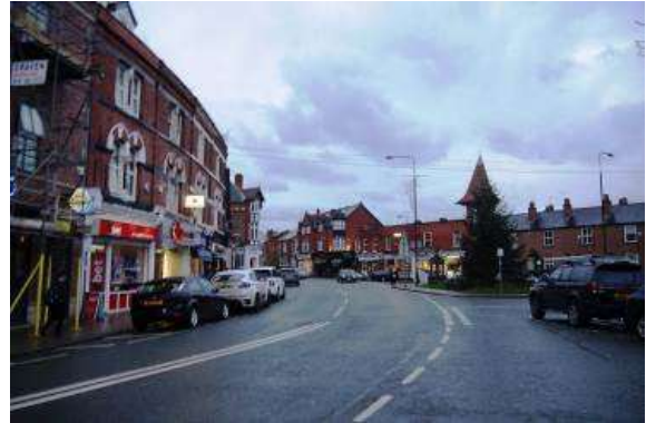
View west along Ashley Road beyond the station
