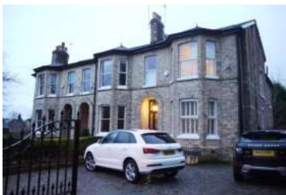
Annex extension to No. 78 Ashley Road
