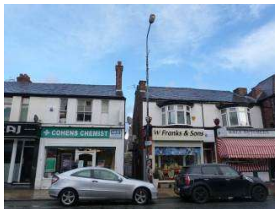
Example of inappropriate fascias and signage along Ashley Road
