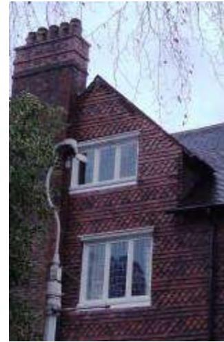
Arts and Crafts details such as chimney stacks, tile-hanging and leaded glazing
