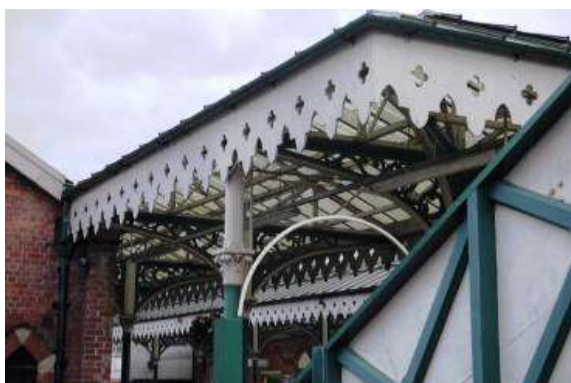
Detail of the east platform canopy
