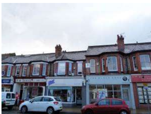
Ashley Road, to the east of the station
