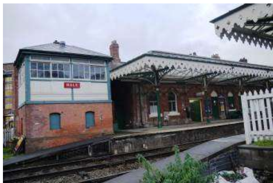
The listed west platform and signal box
