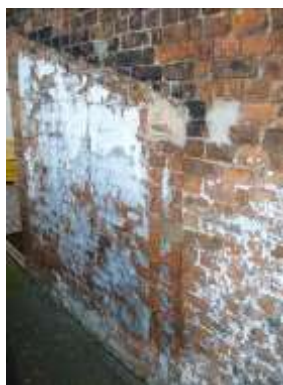
Paint to Vet's brickwork where lean-to has been removed
