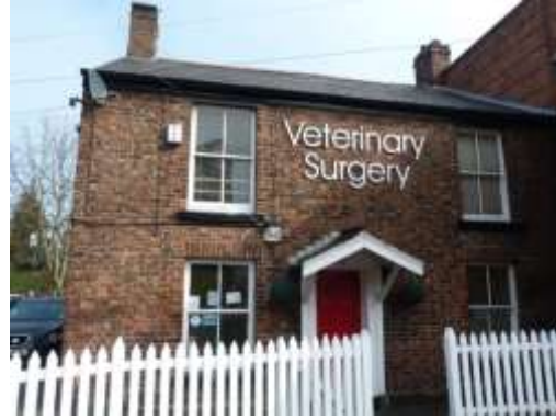
The listed Station Master's House
