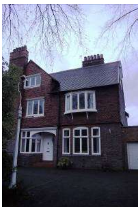
No. 103 Ashley Road, a positive contributor to the Conservation Area
