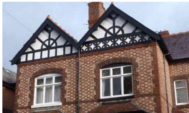
Flemish bond brickwork and timber-framing
