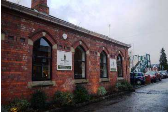
The listed waiting room on the east platform
